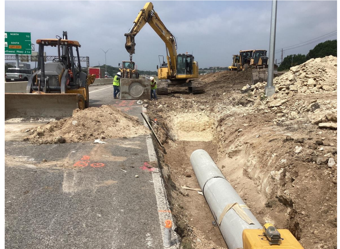
Barton Skyway Entrance Ramp June 2023
